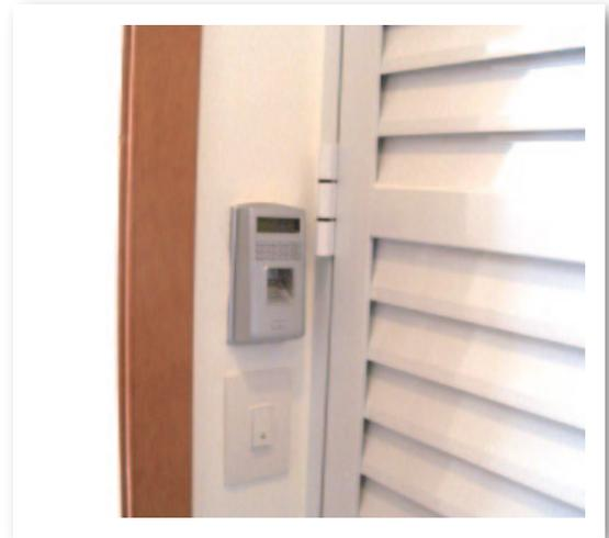
Anviz support Z-Wave to controlling 100% of the lighting, climate, shades, access control (Biometric T-50 with Wireless Z-Wave protocol Via Wiegand26), Audio, Video and Entertainment, all wireless, integrated and controlled by In wall touch-screen panel, Universal Touch-screen Remote control, In wall keypads and iPad. The builder prepare only a Single gang box with 120Vac for each door, no wires to a central control system,
